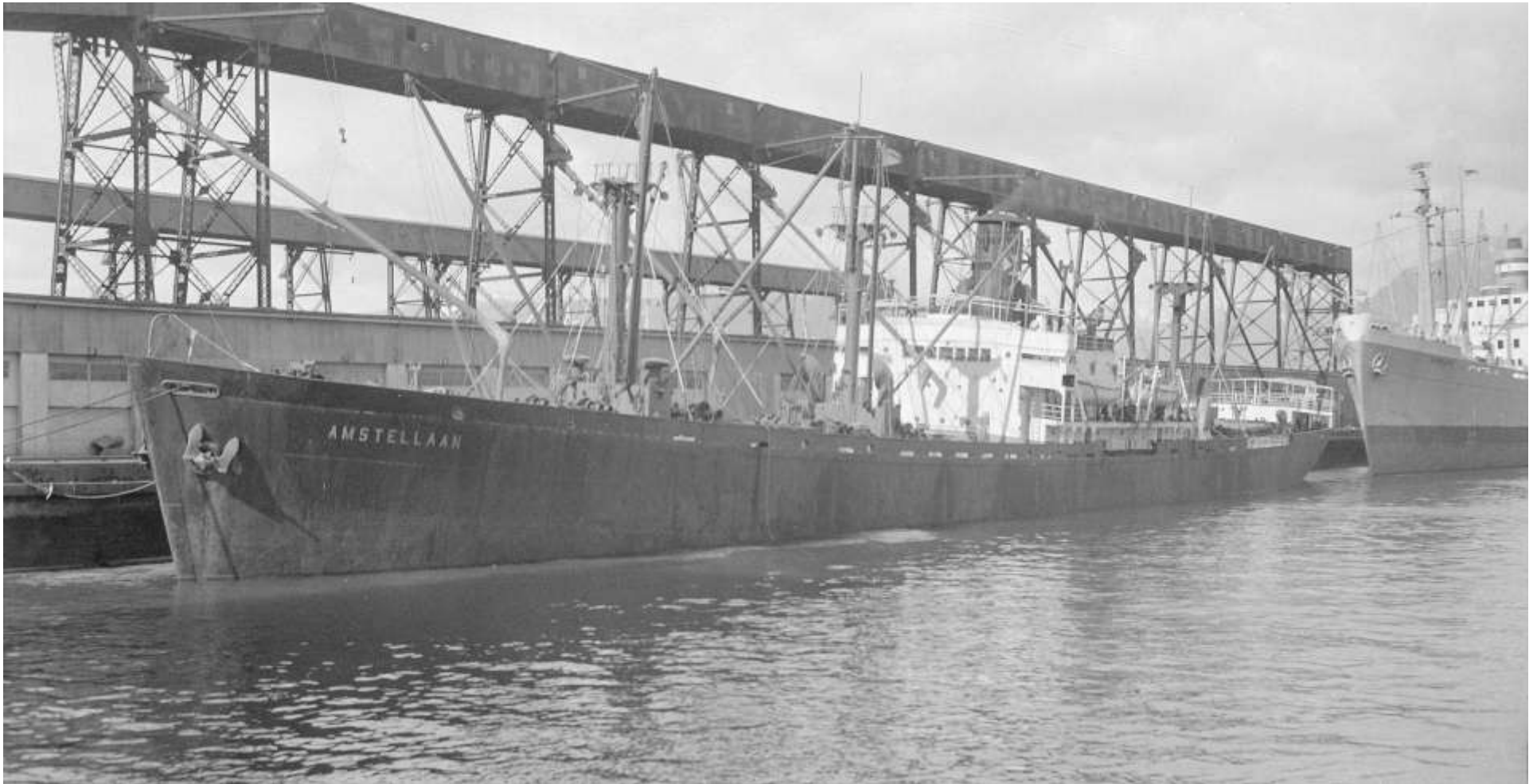
Wheat would be fed into a ship's holds like the Netherlands Steamship Co.'s AMSTELLAAN by the overhead system of conveyer belts and spouts at one of Vancouver's grain terminals such as Lapointe Pier pictured on Wednesday, March 5, 1958 (Vancouver Archives, CVA 447-3116, Photographer - Walter E. Frost)
