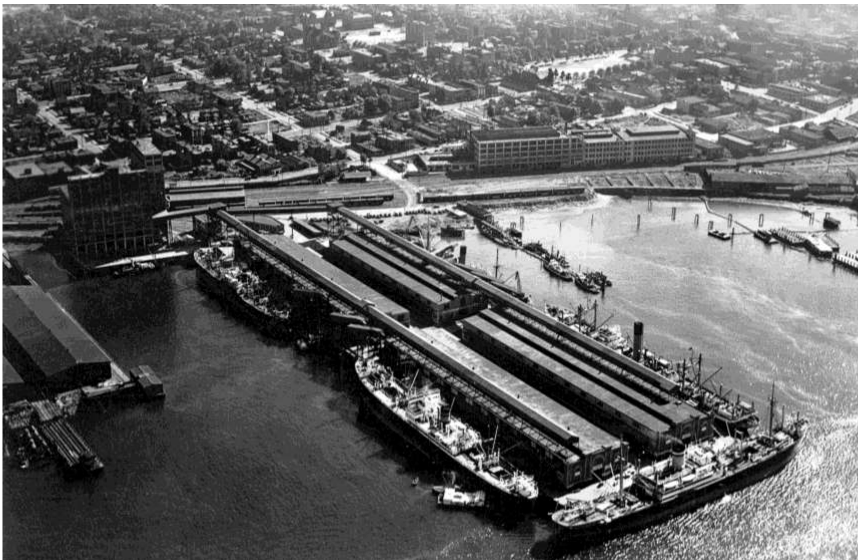
Aerial view of Ballantyne Pier with five sea-going vessels - including two Blue Funnel Line freighters on the far side - taking on grain or discharging / loading breakbulk cargo. Note the covered conveyor belts along each side of the pier connected to VHC Grain Terminal No. 2. (Vancouver Archives, CVA Air P29.4, Major Mathews collection)
