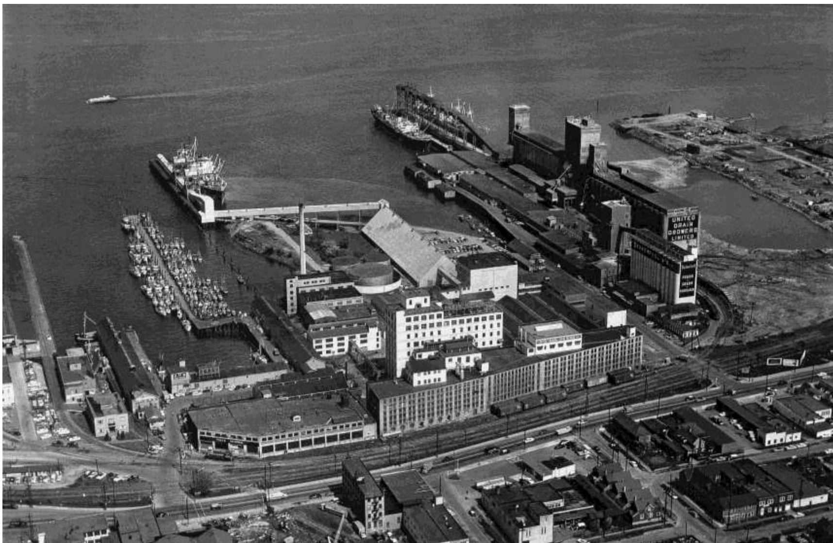
Detail of B.C. Sugar Refinery aerial in 1957 showing the pier, conveyor belts, and storage warehouse (centre) at Rogers Dock. The VHC fishing dock is to the left while to the right are the elevators of today's Alliance Grain Terminal. (Vancouver Archives, CVA 2011-092.3678, B.C. Sugar Museum collection)
