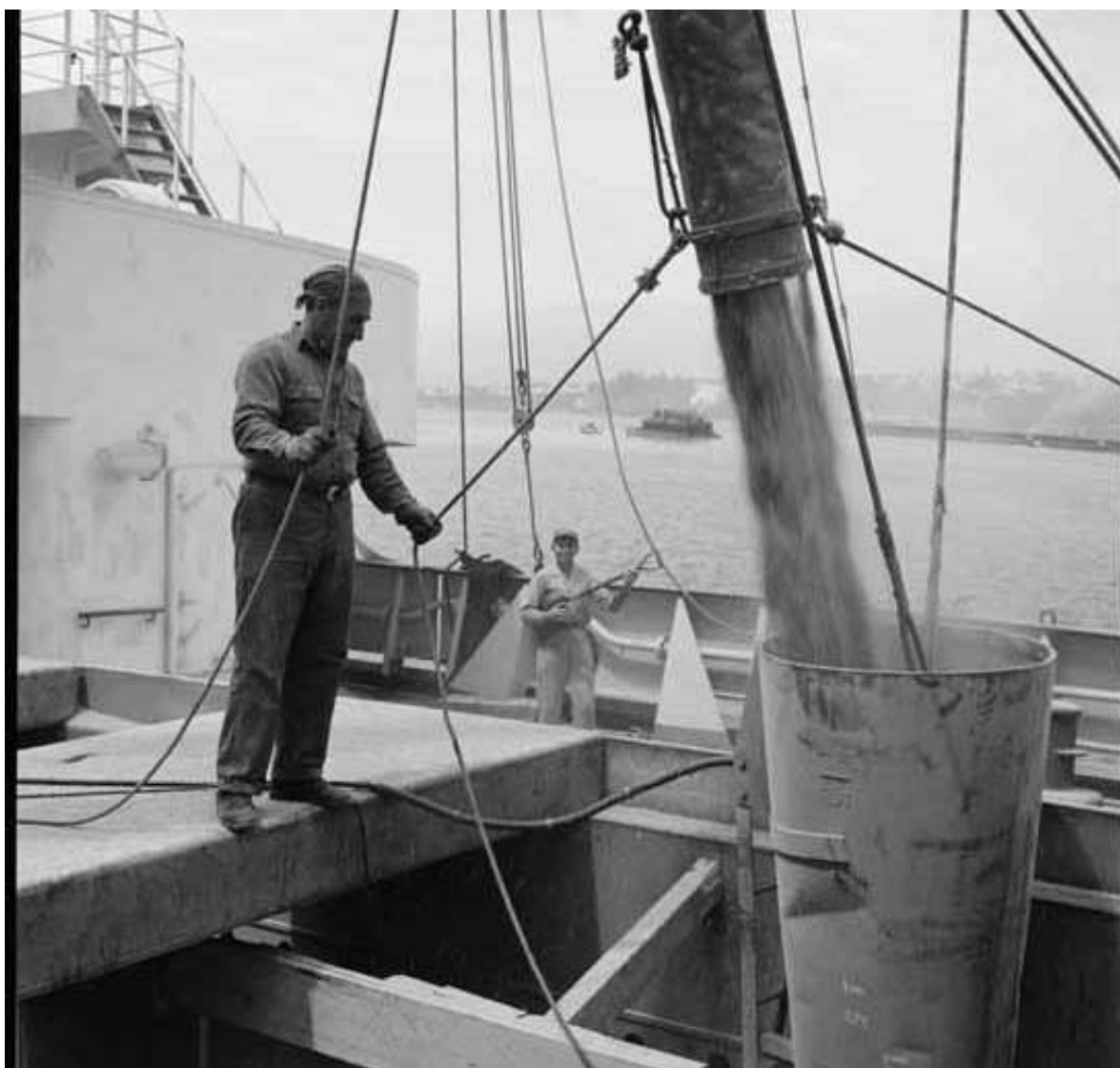
A longshoreman loading wheat on a ship using a mobile shiploading chute at the Alberta Wheat Pool elevator in 1962. Note the longshoreman “playing” the shovel in the background. (Vancouver Public Library, VPL-85781J, Photographer – Stanley Triggs)
