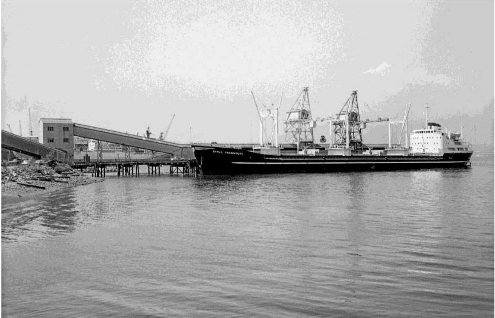
Unloading raw sugar from the MS Stove Transport using the traveling cranes with clam-shell buckets and covered conveyor belts on August 2, 1963.
