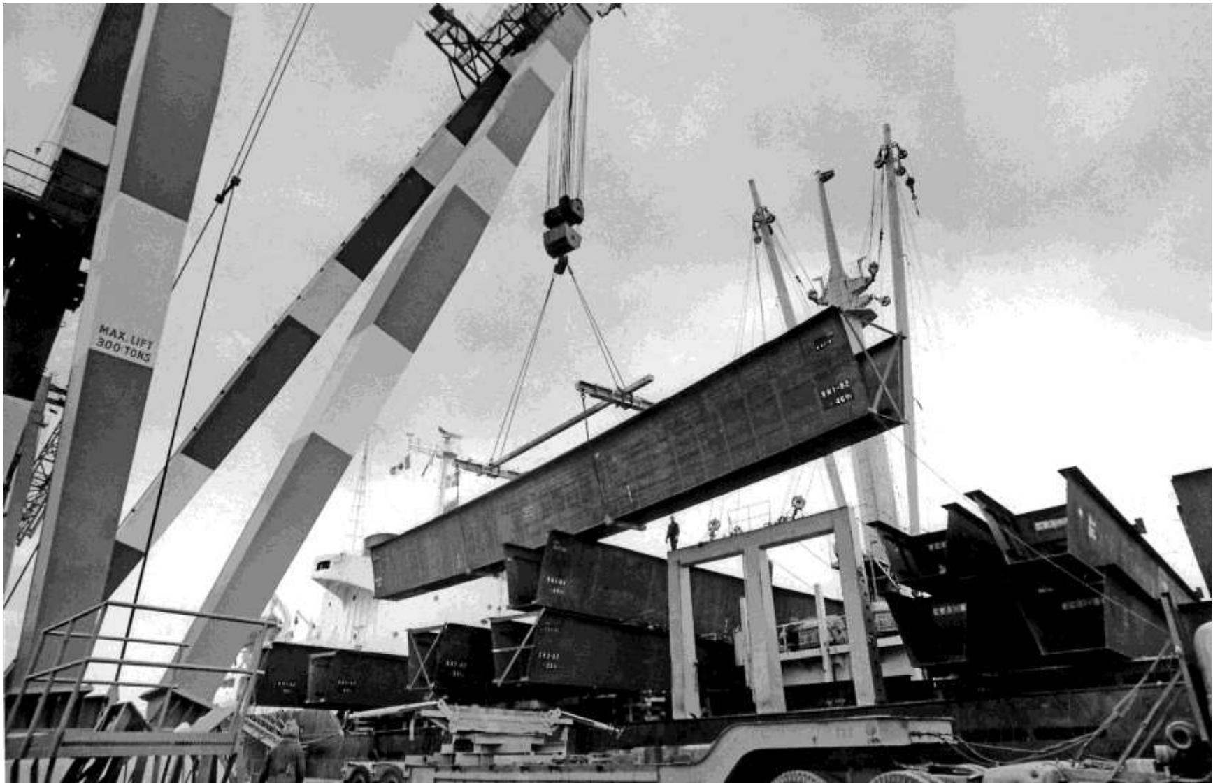
Centennial Pier's 300-ton heavy lift crane unloading 145 ft, 90-ton curved steel beams for use on Portland freeways from the Japanese freighter MS Spruce at Berth 5 on May 6, 1970. (Vancouver Archives, CVA 134-190, Pugstem Publications)
