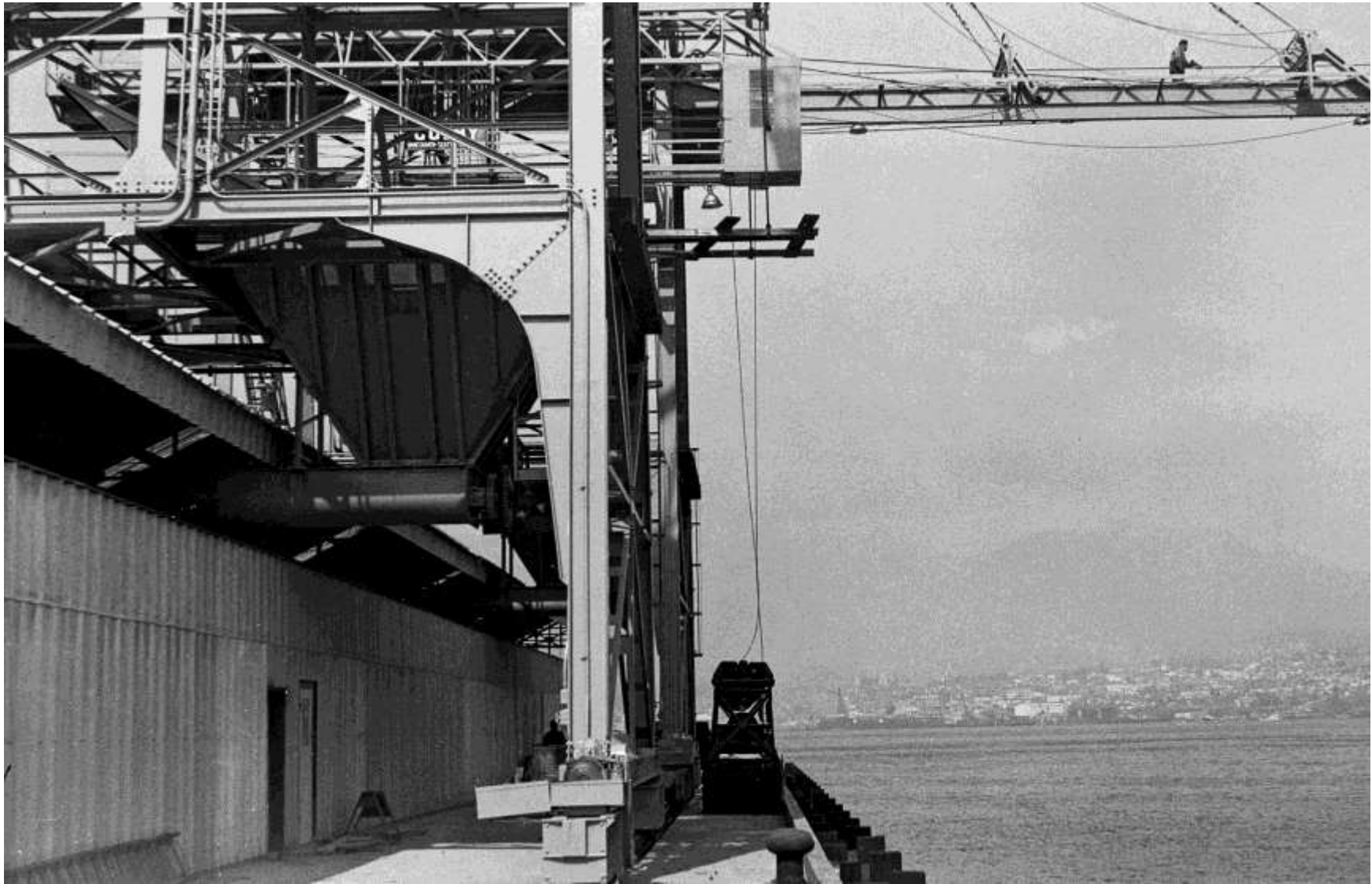
Automation using travelling cranes, clam-shell buckets, hoppers, and covered conveyor belts changed the discharge of raw sugar from a breakbulk (bags manually unloaded by longshoremen) to a bulk commodity that was faster and cheaper to discharge. (Vancouver Archives, CVA 2011-092.2797, B.C. Sugar Museum collection)
