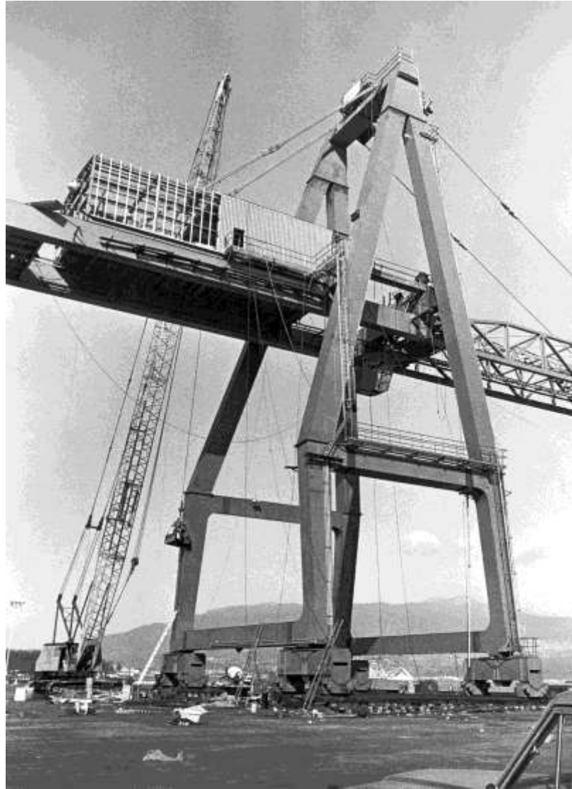
Massive metallic monster - Port of Vancouver's new quay crane for containerized shipping nears completion at Centennial Pier on March 7, 1970. The crane, which is first of its type in Vancouver harbour facilitated easy handling of shipping containers. (Vancouver Archives, CVA 134-022, Pugstem Publications)
